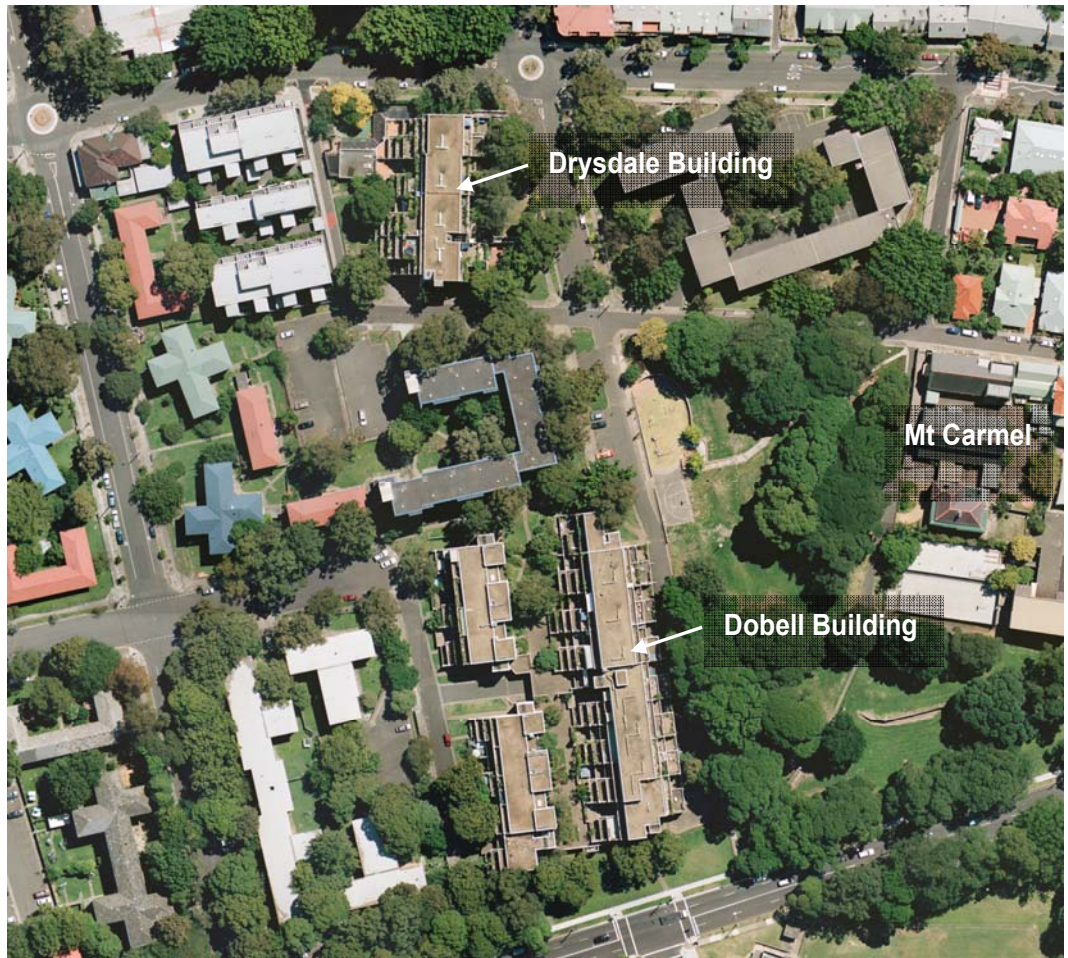
Figure 27. Drysdale and Dobell aerial view. These buildings may be capable of green roofs.
