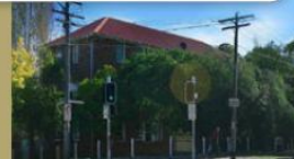
Redfern East Development
