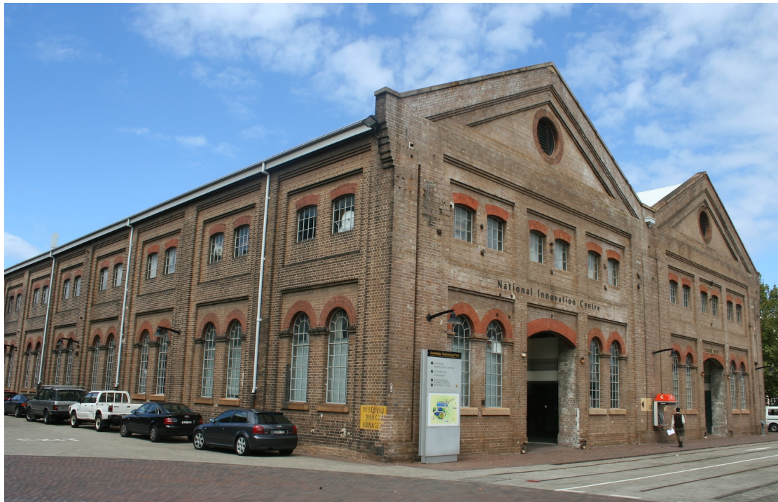
Figure 4 - the National Innovation Centre (north facade)
