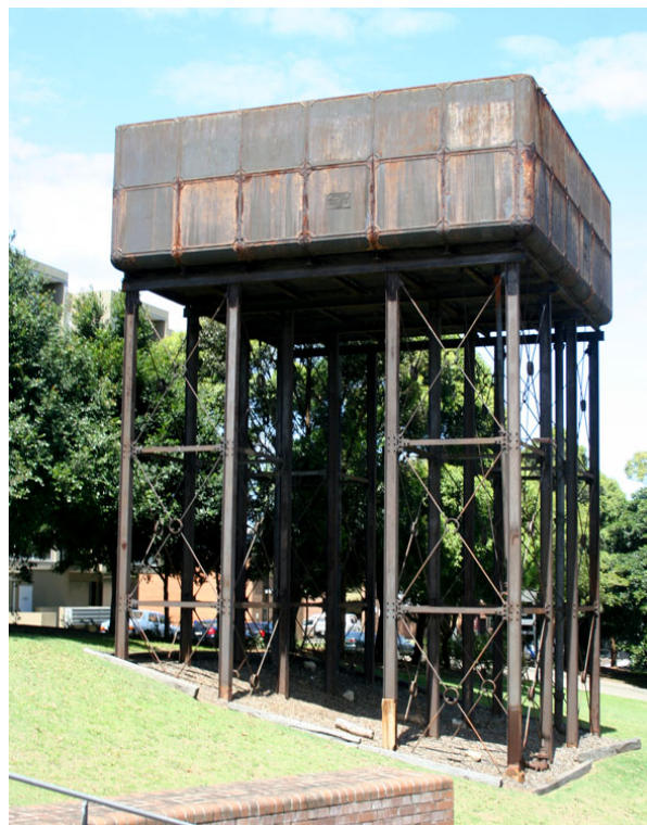
Figure 6 - The Water Tower (north elevation)
