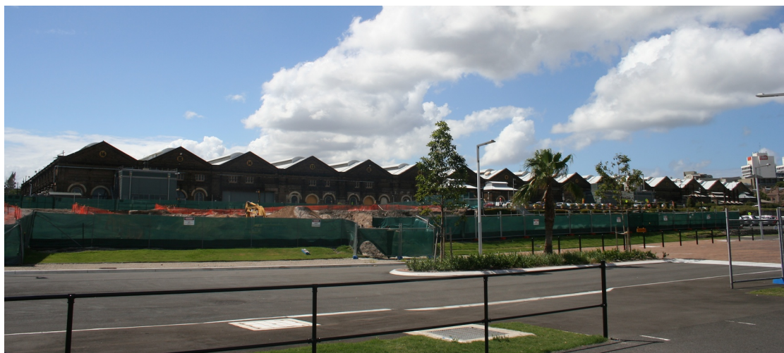
Figure 3 - The Locomotive Workshops (south facade)
