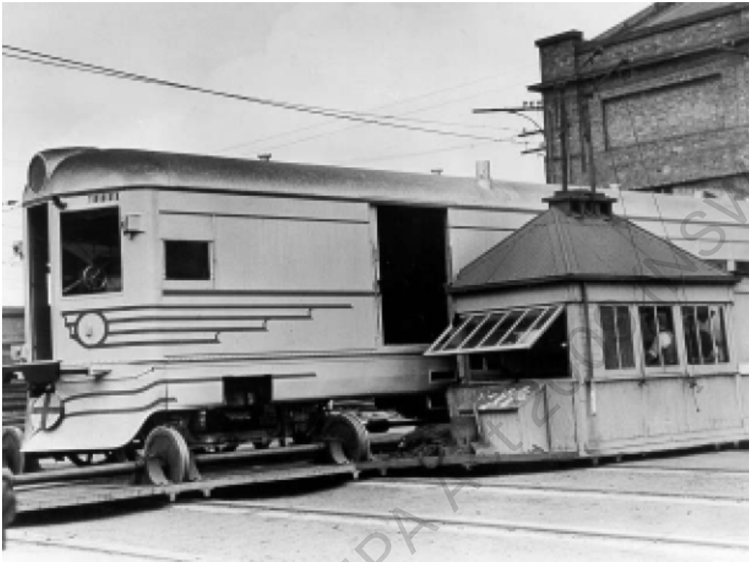
Figure 1.9: Traverser No.1 at the Eveleigh Carriageworks c.1937 carrying a 400 class Rail Motor (Source: SRAO)
