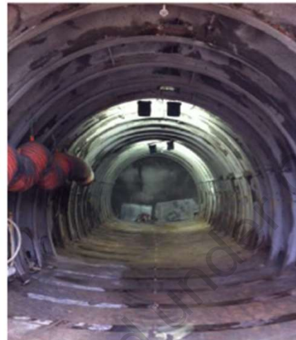
Image from the Arncliffe Pedestrian underpass, completed 2.5m below running rail
