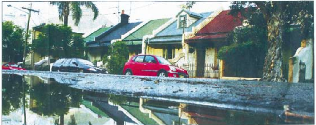
Uncertain future ... a row of houses on Leamington Avenue, Newtown, that RailCorp is thinking of demolishing. Photo: Dallas Kilponen
