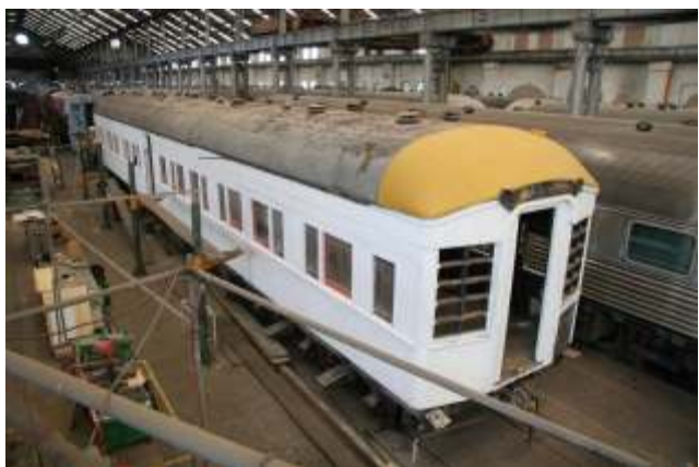
Completely new side and end panels fitted
