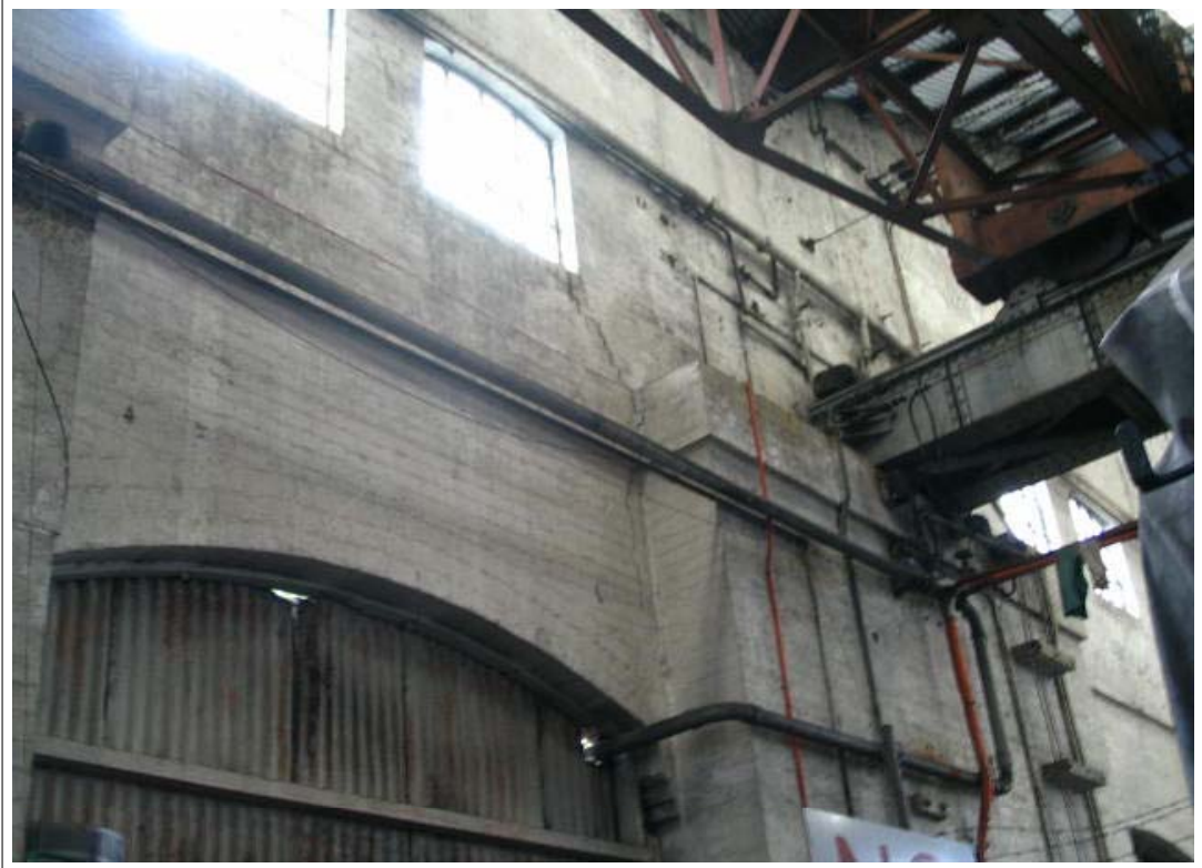
25 Stepped cracking to right hand side of rear gable window.
