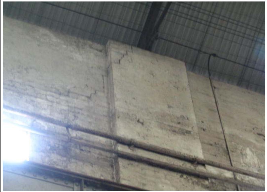
23 General high level cracking to South wall.
