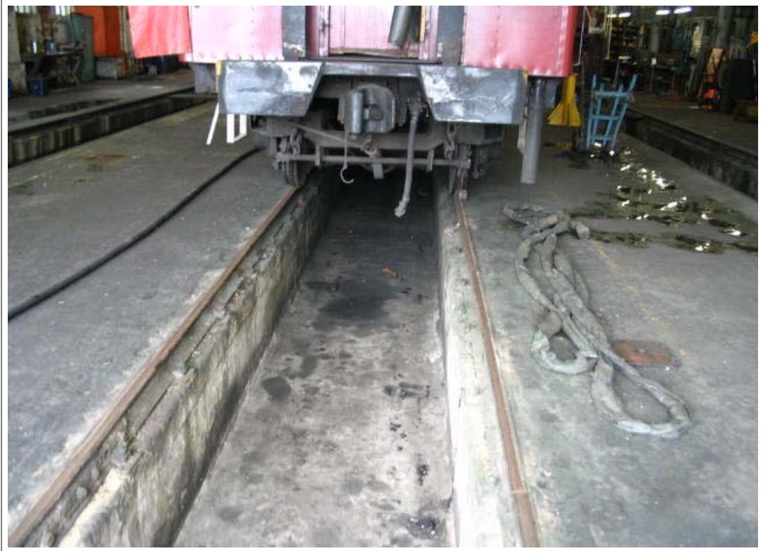
17 Open internal inspection pits.
