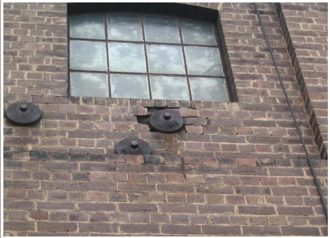
29 Brickwork repairs required around crane restraint fixing.
