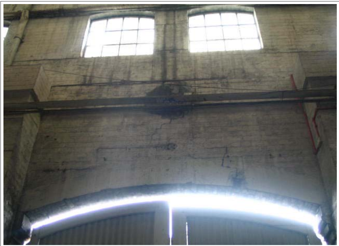
24 General cracking over Eastern rear gable wall.
