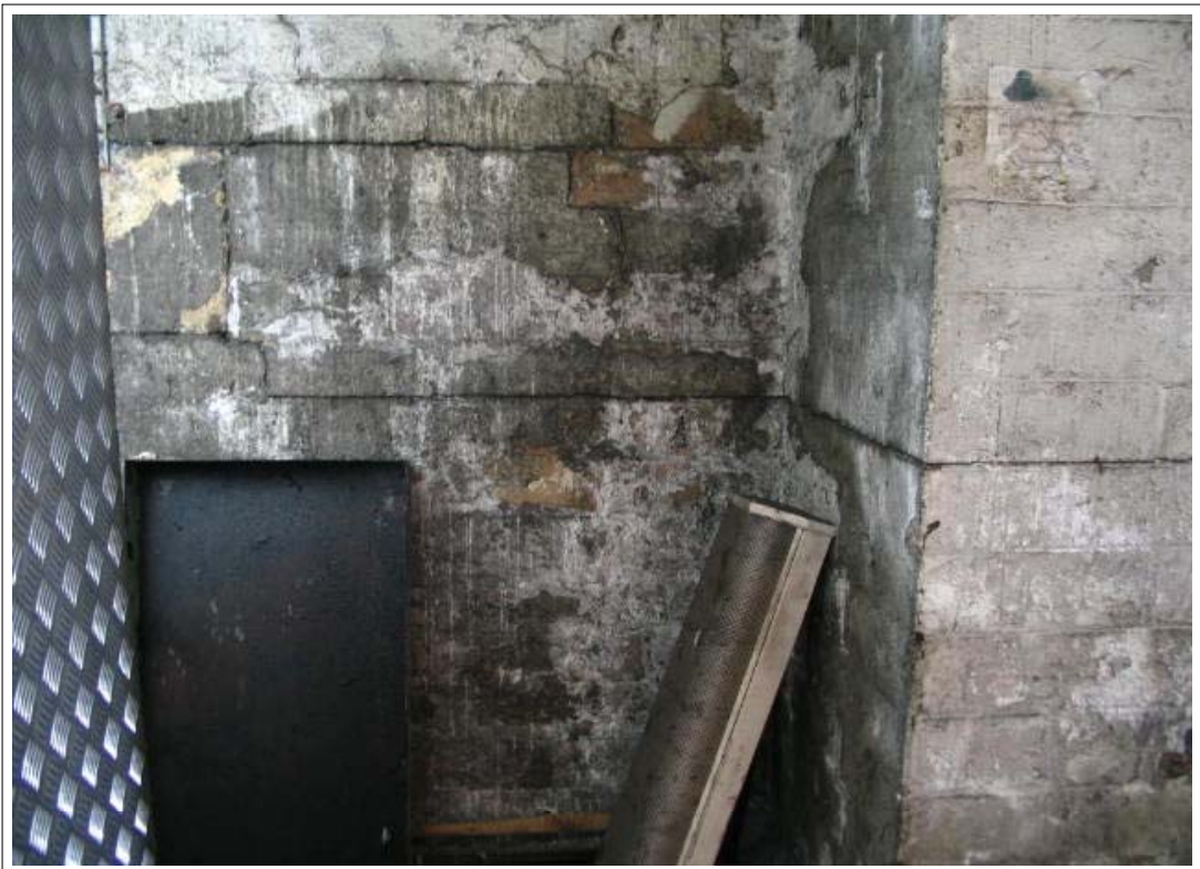
22 Low level internal horizontal crack line to Southern wall.
