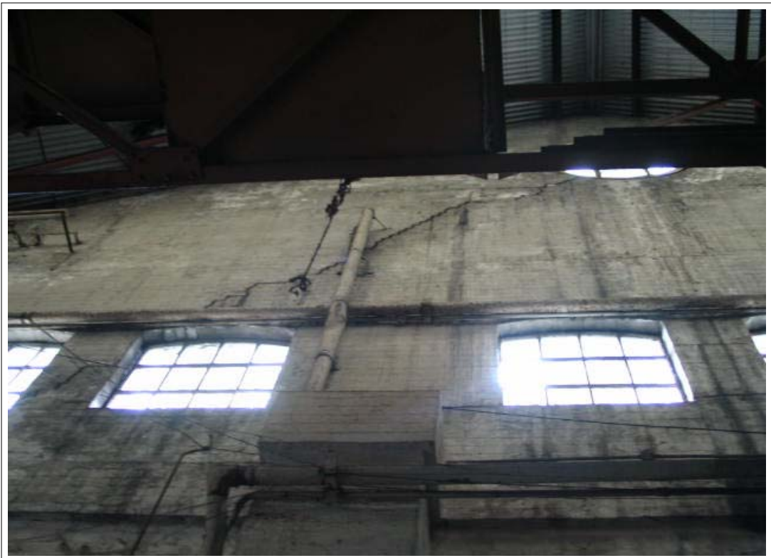
26 Large stepped crack to rear eastern gable wall.
