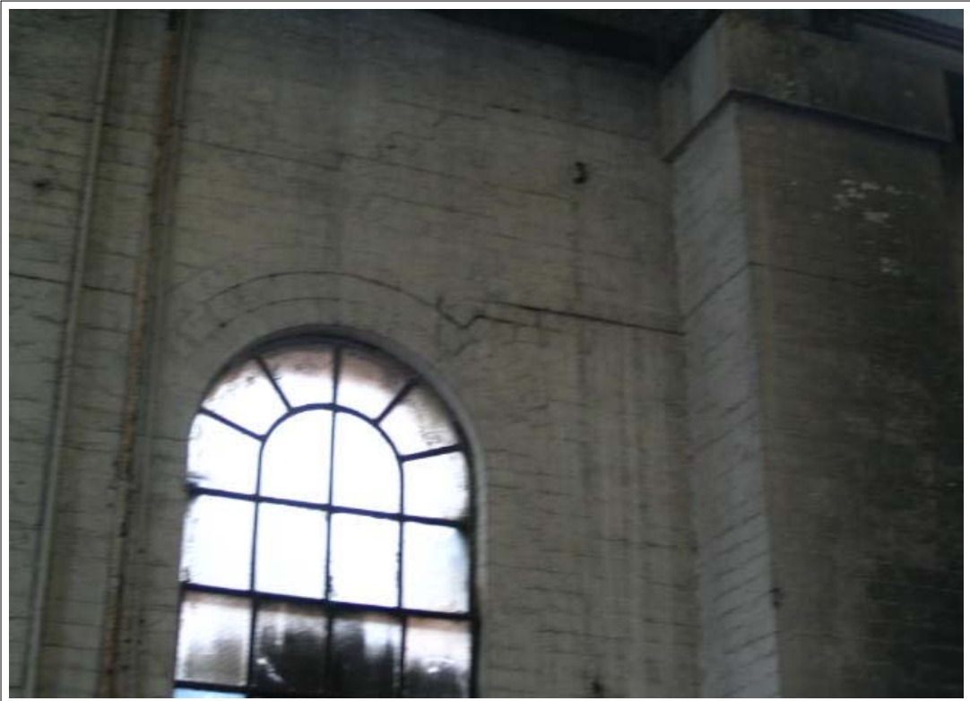
28 Horizontal cracking to the head of the window to the northern wall.
