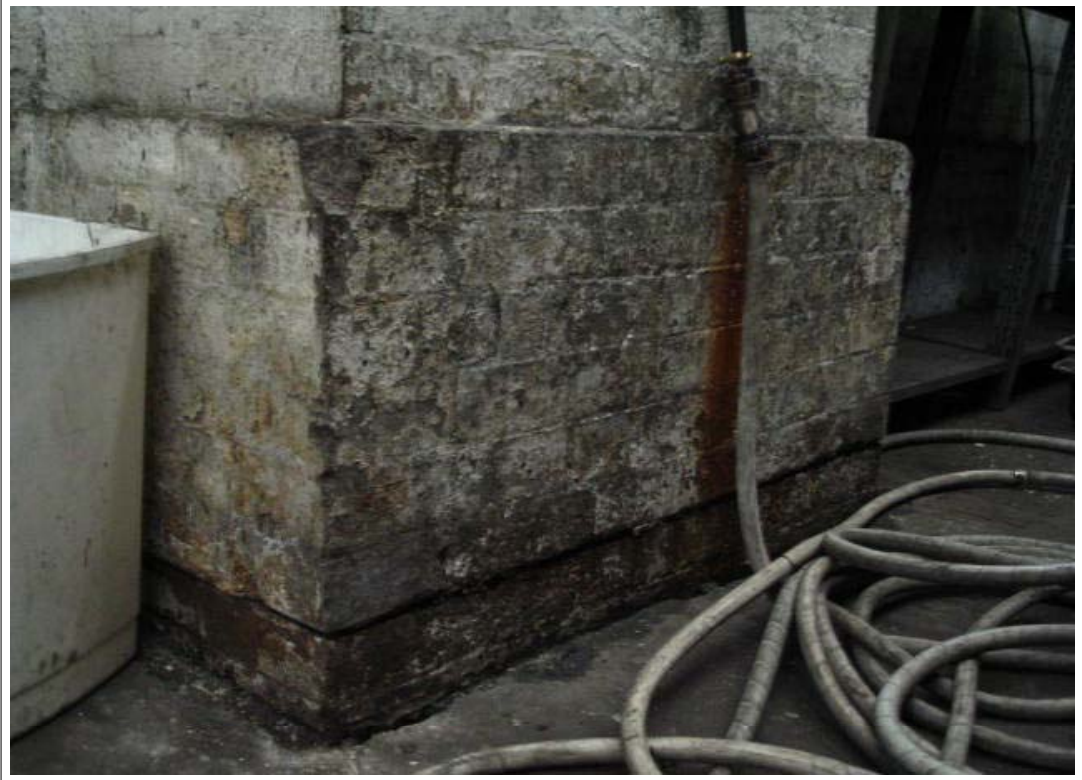
27 Horizontal cracking / minor displacement on damp proof course line.
