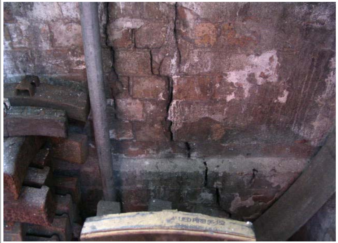
21 Internal cracking to bay 1 of the Southern wall.
