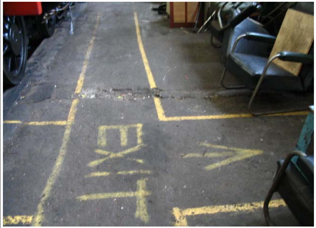
33 Floor slab displaced around service conduit.
