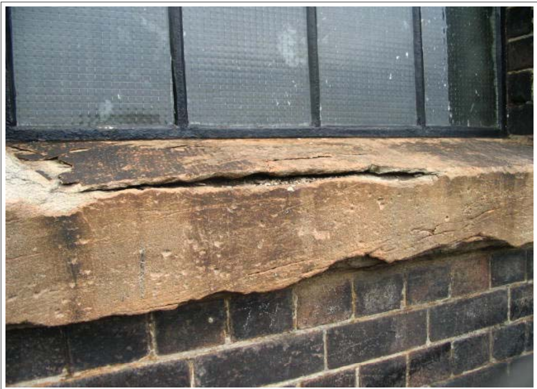
30 Spalling stone window sub-cill.
