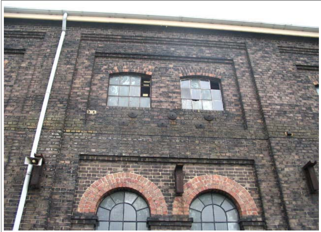
7 South elevation. General missing window panes.
