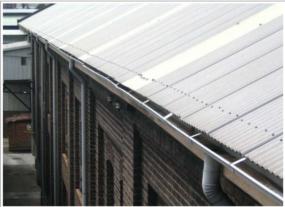
12 Roof gutter requires realignment.
