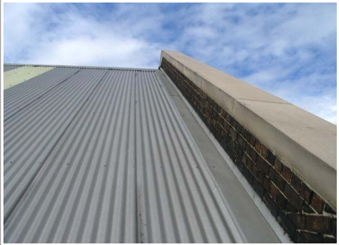
11 Roof flashing in good order.
