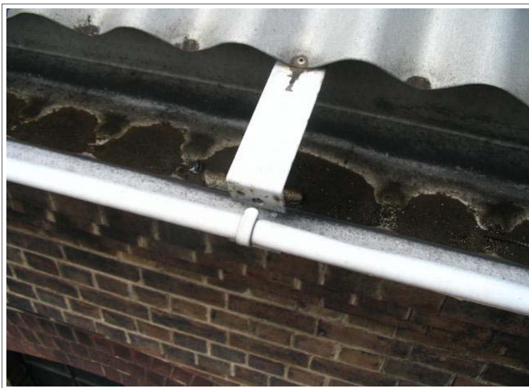
20 Broken gutter fixing bracket.
