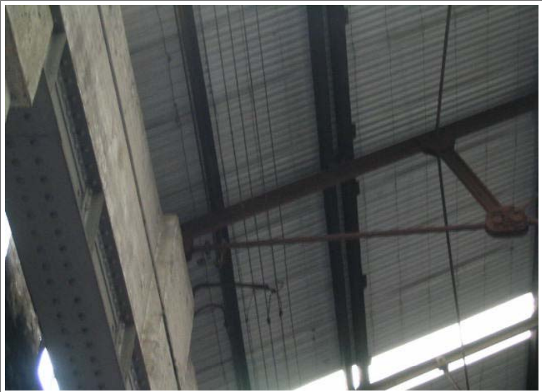
14 End truss to North side. Note exposed electrical cables and slender bottom truss rod.
