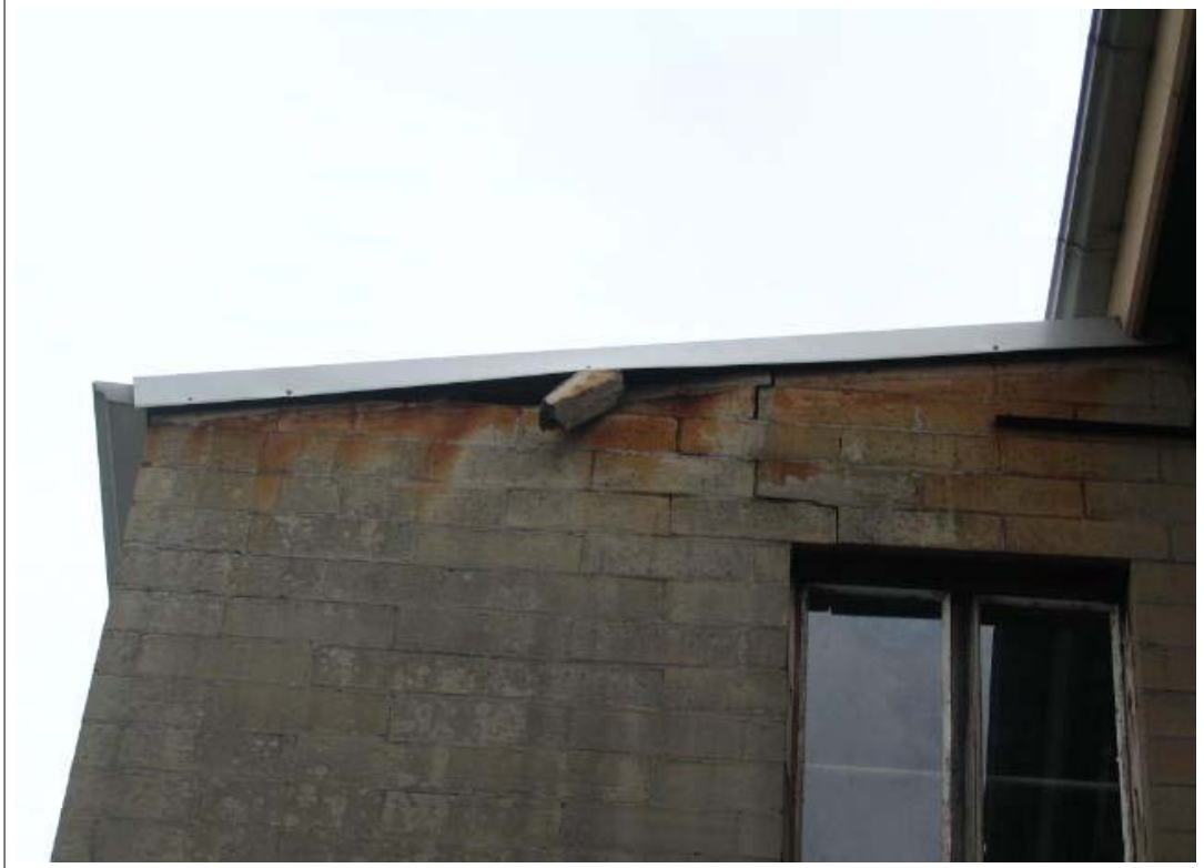
31 Loose block to South elevation.
