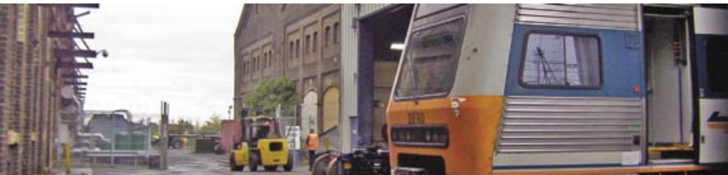
South Eveleigh - Xplorer Endeavour Service Centre and Large Erecting Shed in the background
