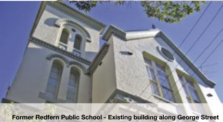
Former Redfern Public School - Existing building along George Street
