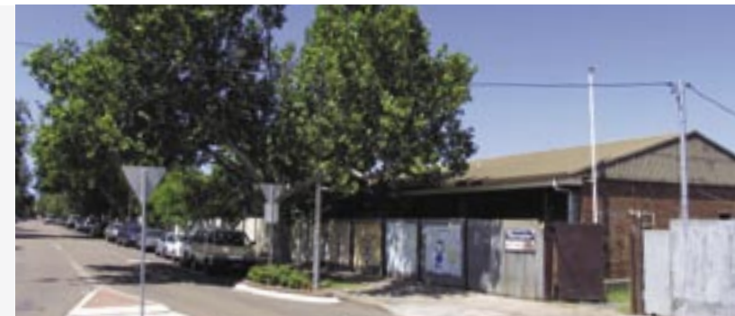
Existing - Former Canteen and Construction building off Wilson Street
