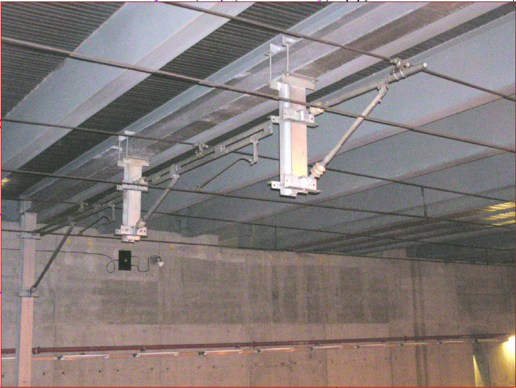
PHOTO 1. THIS PHOTO SHOWS A PORTAL STRUCTURE UNDER A CONCOURSE STRUCTURE WITH A 5.2 METRE MINIMUM CLEARANCE (MELBOURNE)
