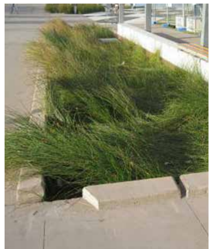
RAINGARDENS Filtering stormwater
