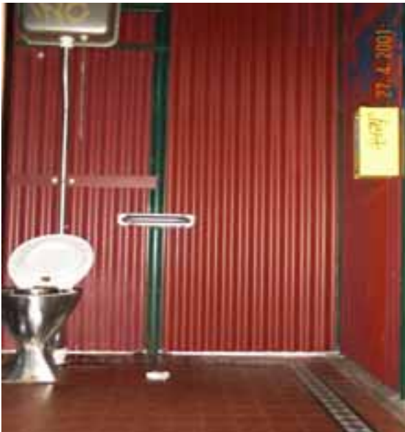
A fixed syringe bin in a public toilet part of Council's commitment to the safe disposal of needles and syringes.
